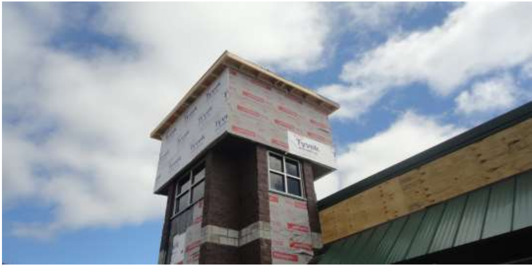
2018 Amended Application. Photos of work in progress. North tower.
