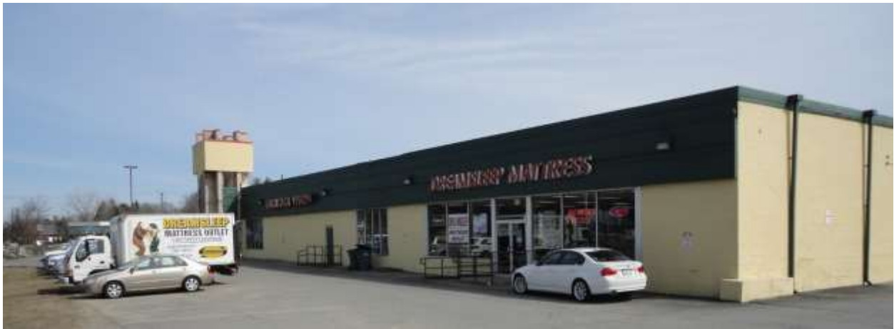
Existing Rte. 29 façade, northwest corner.
