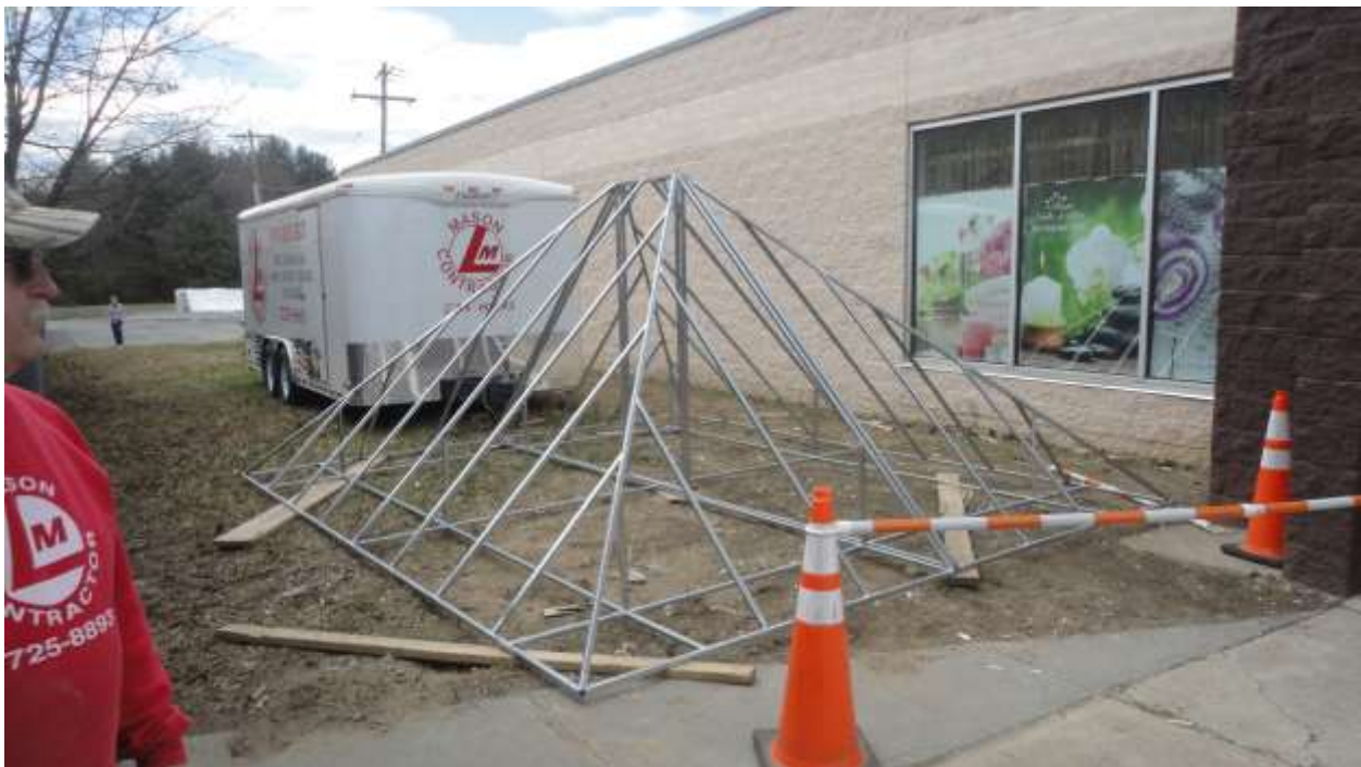
New tower roof structural aluminum tube frame.
