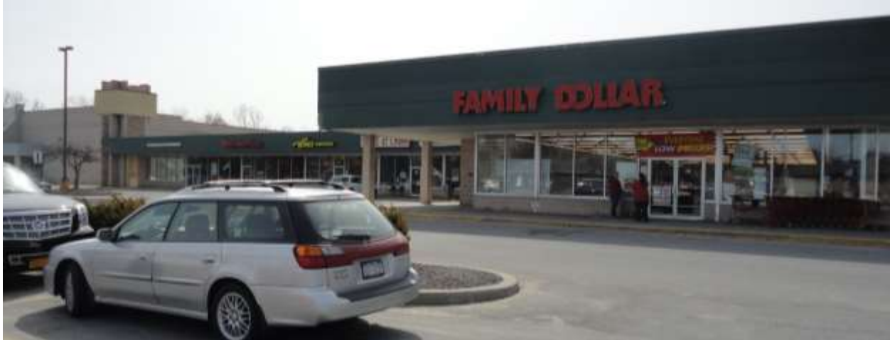
Existing West Ave. façade showing covered sidewalk.
