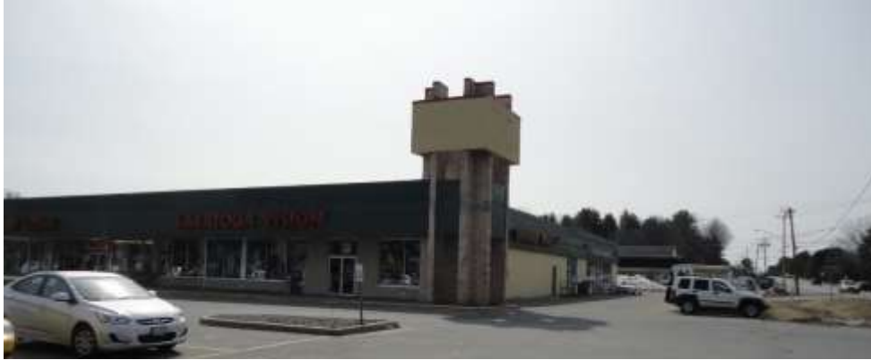
Existing corner tower facing Rte. 29 & West Ave.
