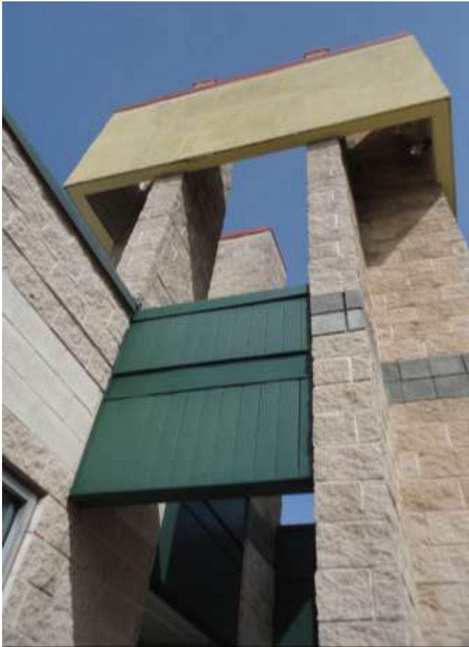
Existing tower detail.
